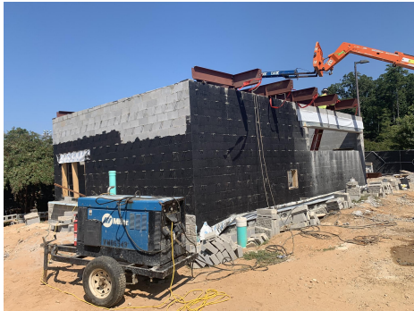
CSK- Concession structural steel installation
