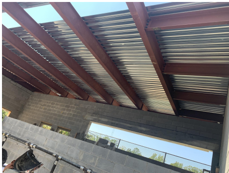
CSK- Concession steel deck installation
